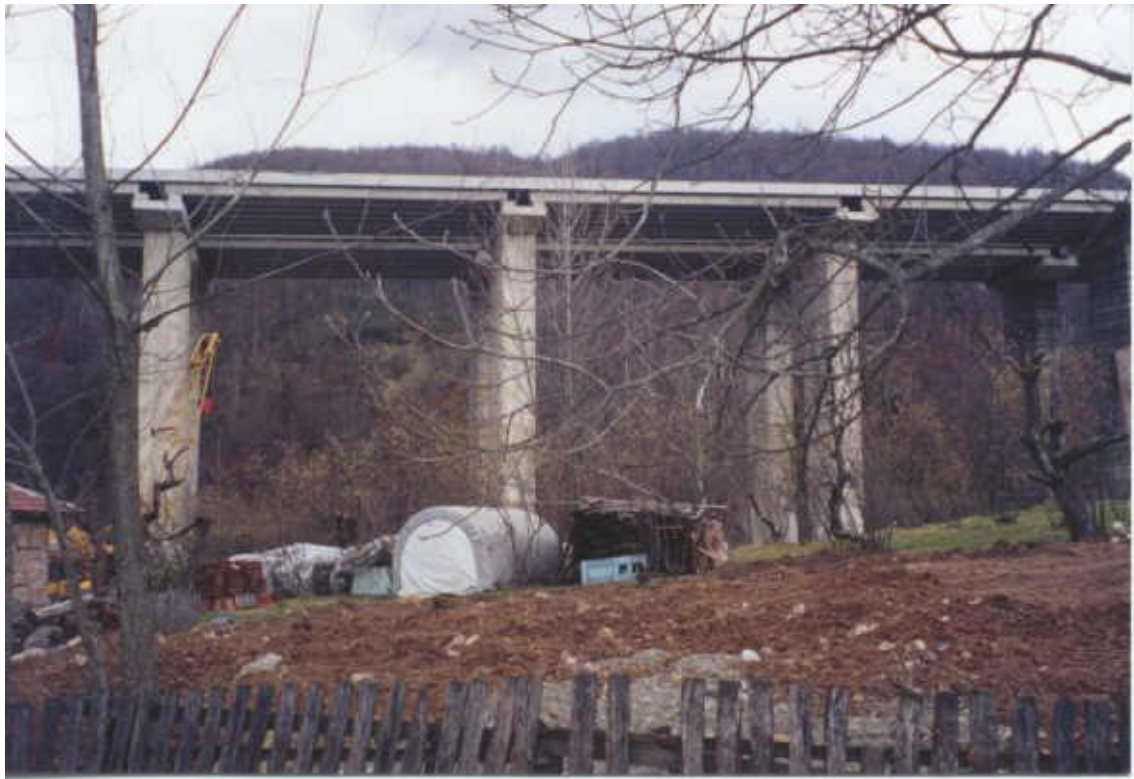
Fig. 1, – Two photos showing general views of the viaduct.
